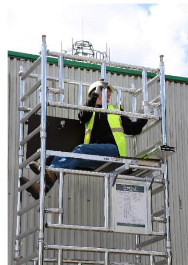
29. Fit 2 guardrail frames, with the top hook (facing outwards) set above the top rung of the frame.
