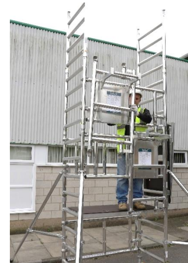
25. Retrieve a side guardrail frame from the front assembly bracket and locate it as shown.
